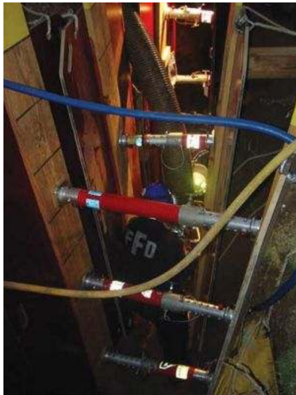
(5) The rescuers remove soil from the victim with the rescue vacuum and the air knife
