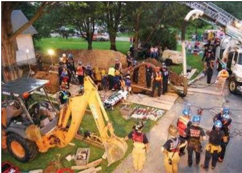
(3) HCTRT members operate the rescue vacuum system.
