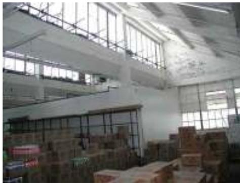
(5) Northern light from a sawtooth roof uniformly illuminates the interior space.
