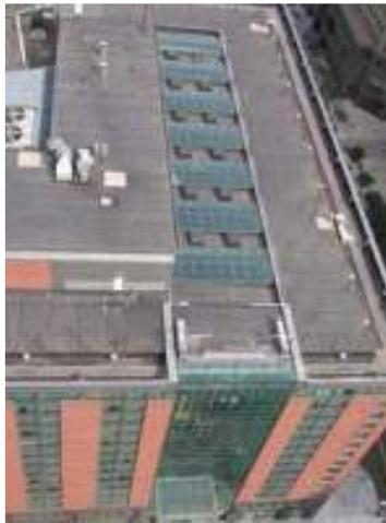
(4) A rooftop view of Embassy Suites reveals a comprehensive layout of atrium skylights and ventilation hatches. Chief officers should know how these features are controlled and operated automatically and manually by building maintenance engineers.
